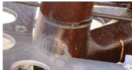
Diamond Wire Cutting
